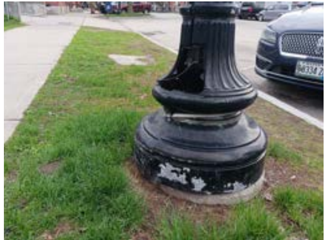
Light Pole Base
