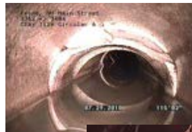
Sewer Infrastructure Condition
