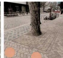
Interlocking units with permeable aggregate joints
