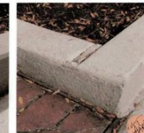
Cast-in-place concrete curb
