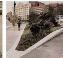
Precast concrete - flush curb to seat wall transition
