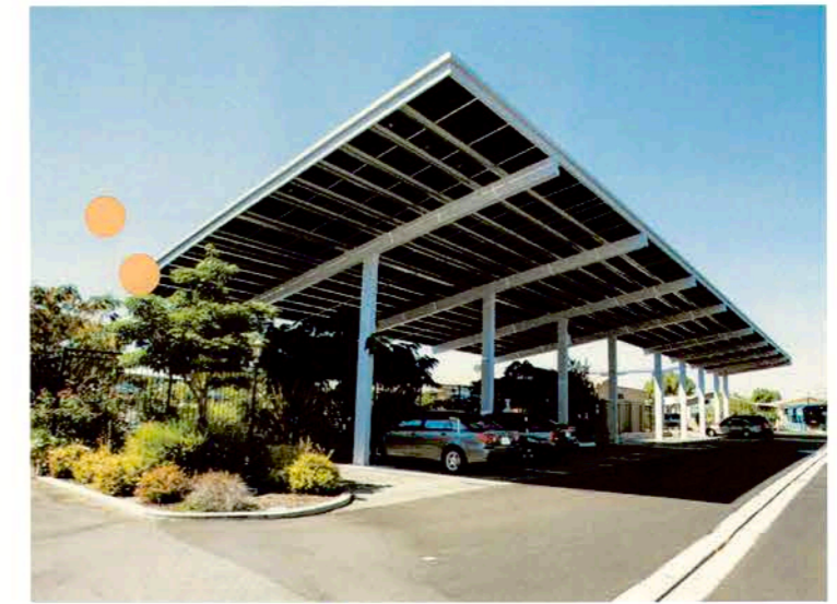
Solar Structure over Parking
