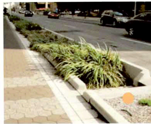
Bioswale separates sidewalks from bike lanes and vehicular traffic
