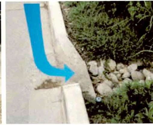
An angled curb cut with a graded
