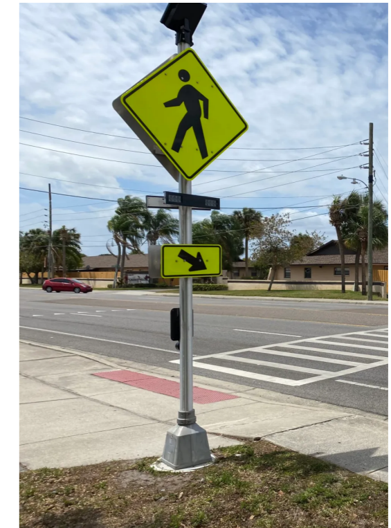
Rectangular Rapid Flashing Beacon
