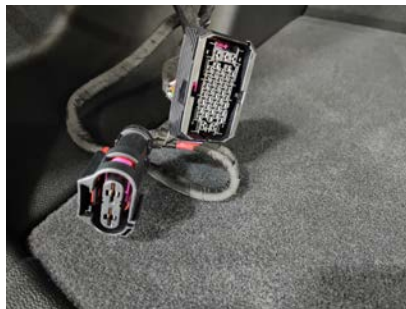
Located behind left rear cargo trim
