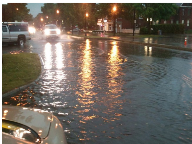
Nuisance flooding at the intersection of Eagle Ct. and Main Street.
