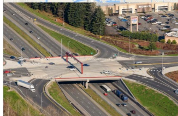
Aerial view of the completed 116th Street NE interchange looking northeast.
