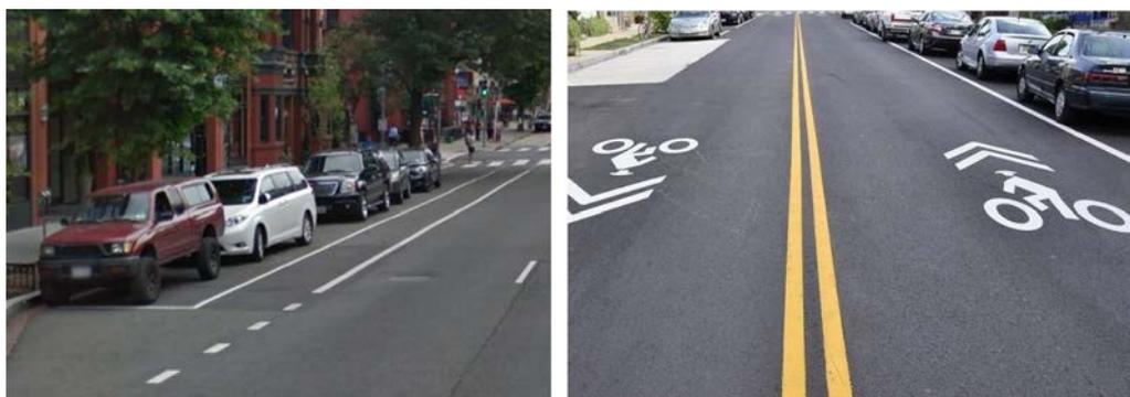
Fig. 1. Examples of a bike lane (left) and sharrows (right).
