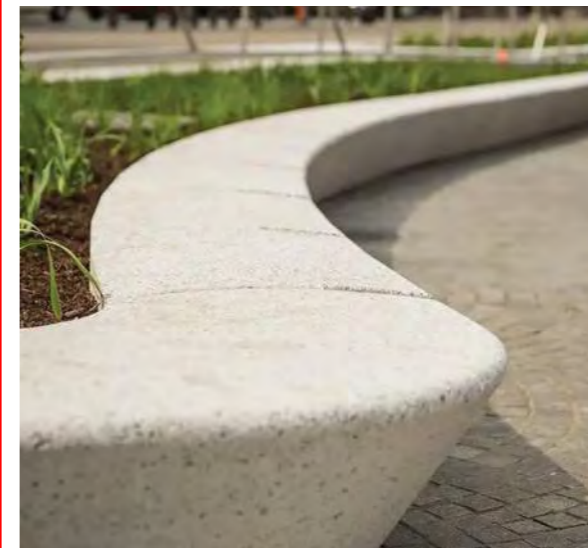
Precast concrete seatwall
