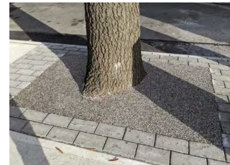
Permeable Resin Bound Paving
