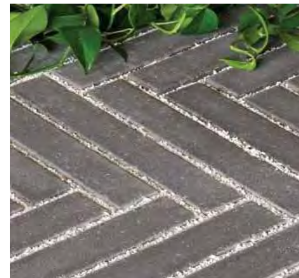
Interlocking units with permeable aggregate joints
