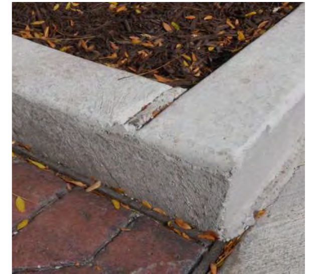
Cast-in-place concrete curb
