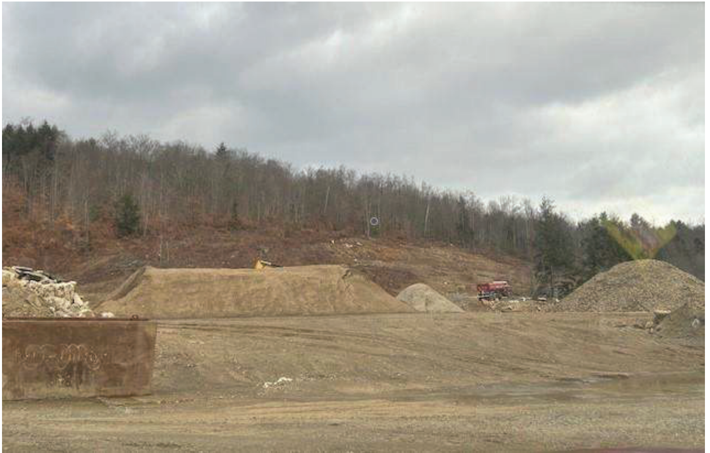
Existing Material and Processing Area, Looking North December 12, 2024
