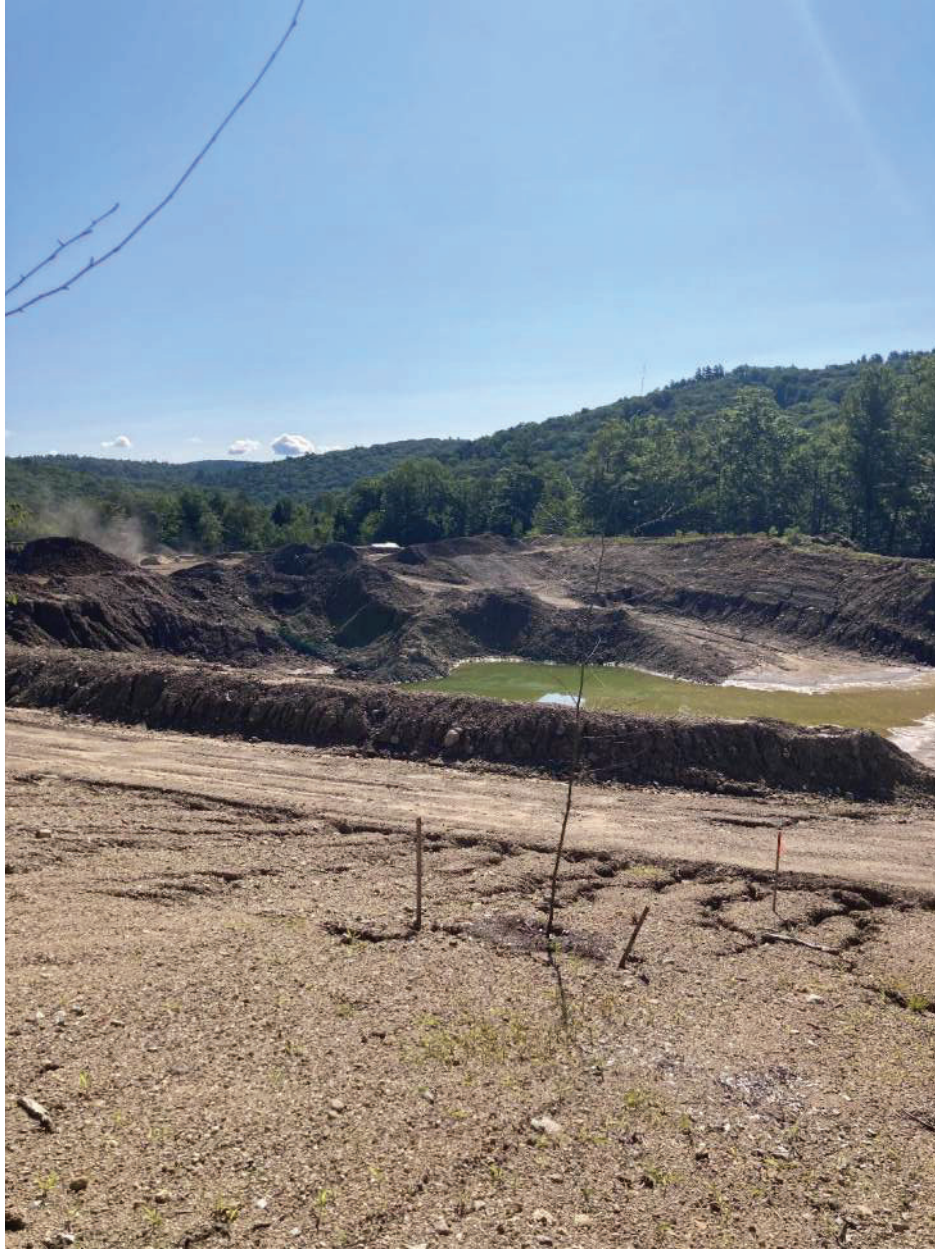
Looking at Current Gravel Operation August 3, 2024
