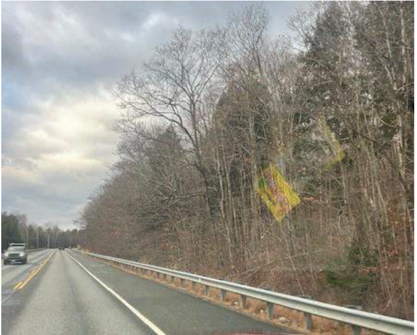
Existing Woodland Buffer from NH Route 9, Looking West December 12, 2024
