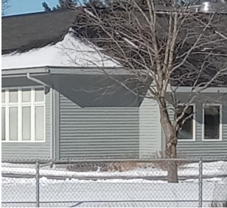
Photo 5: Proposed Inverter and Transformer Location
