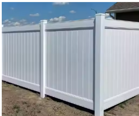
Example vinyl privacy screen for exterior AC equipment
