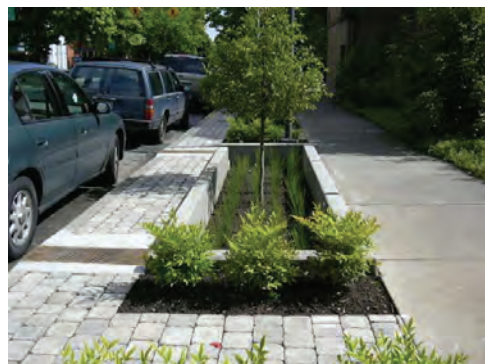
Example of continuous planters to enhance tree health and stormwater management incorporated into the streetscape
