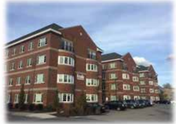
Figure 4.2. Arcadia Apartments. Photo Source: Authors
