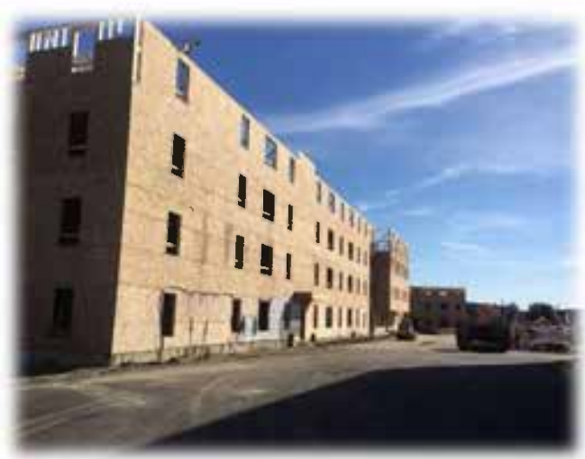
Figure 4.5. Construction of new apartments at Washington Park of Keene LLC. Source: Authors
