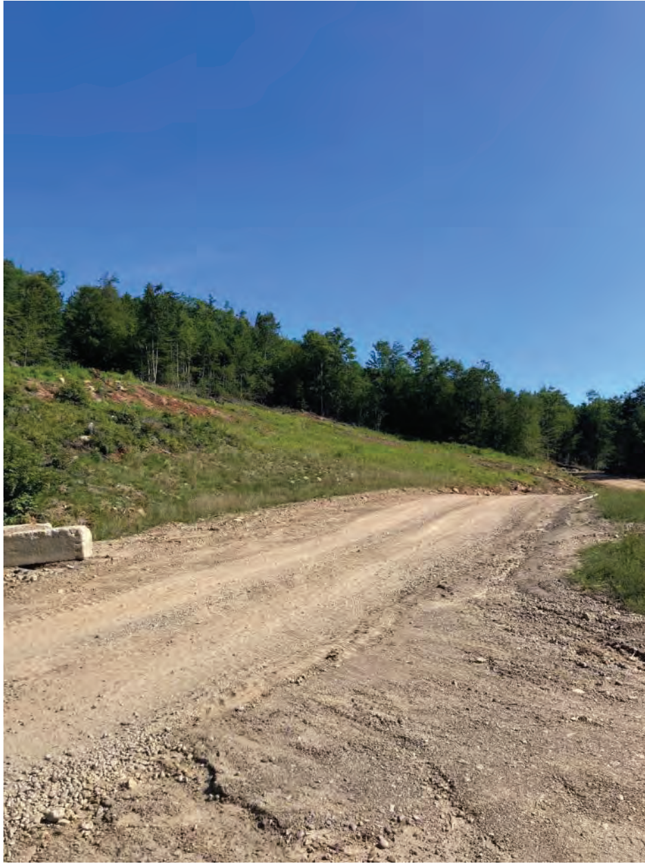
Looking at Existing Logging Road August 3, 2024
