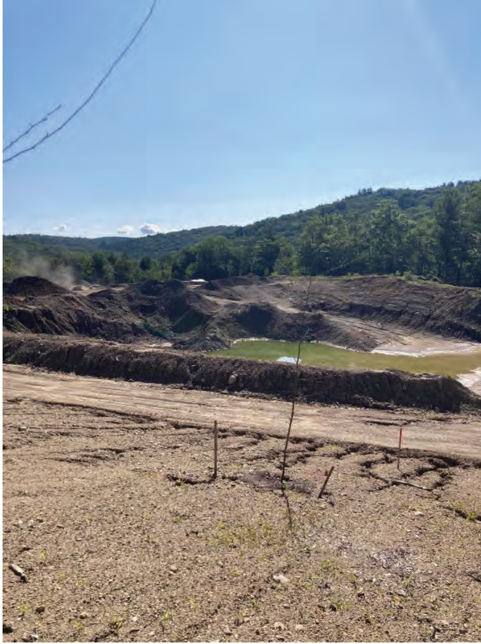
Looking at Current Gravel Operation August 3, 2024
