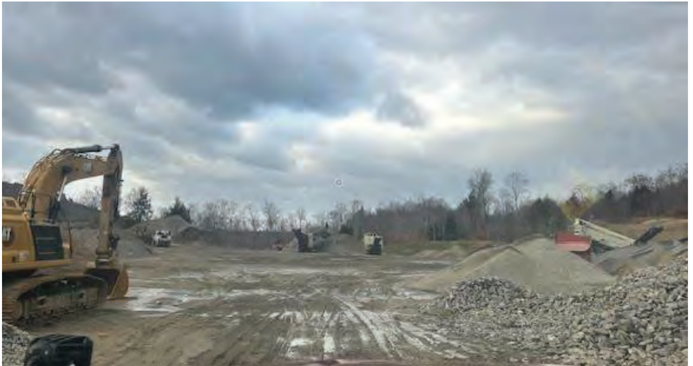
Existing Material and Processing Area, Looking West December 12, 2024
