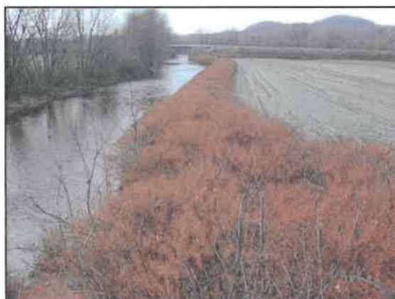
River embankment/floodplain/farm field impacts
