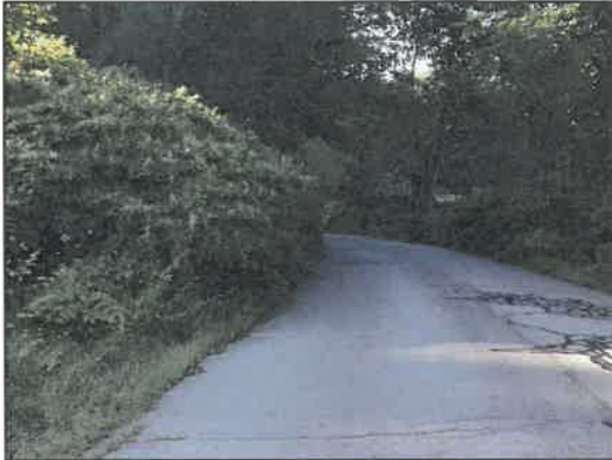
Roadway sight distance and safety issues
