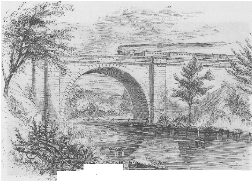
Viaduct of Cheshire Railroad at South Keene
