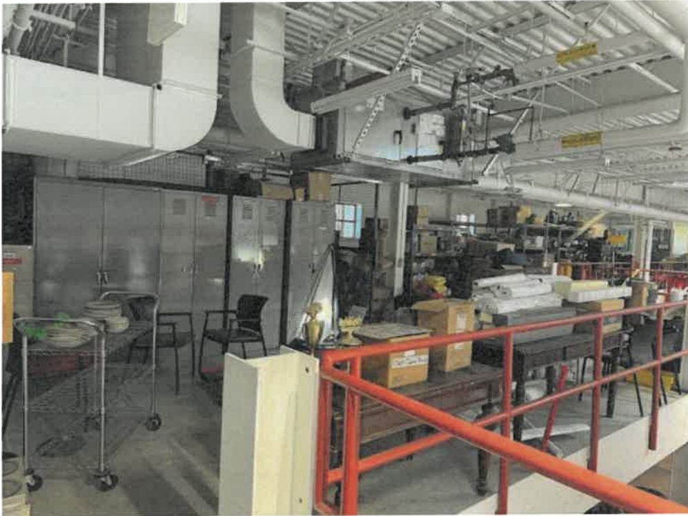
View of mezzanine space currently being used for storage
