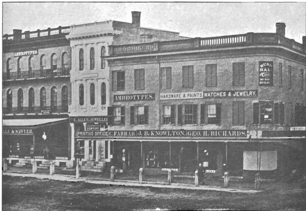
RICHARDS, COLONY AND SHELLY & SAWYER BUILDINGS. DESTROYED BY FIRE IN 1865.
