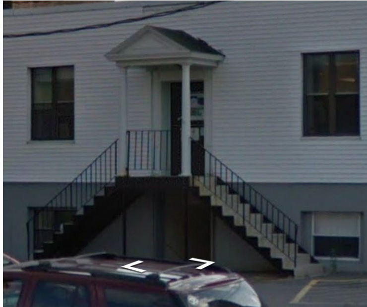
Fig 4: Existing Covered Entryway (To Be Removed)
