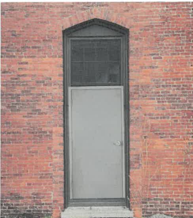
Mockup of door installed in window opening. Door to be painted bronze to match trim.
