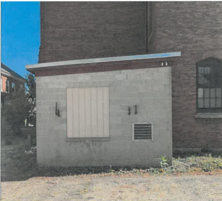
View of Boiler Room from Rear – HVAC Equipment will be placed on the roof and screened with wood louvers to allow air flow to the equipment while masking the equipment from neighboring properties.
