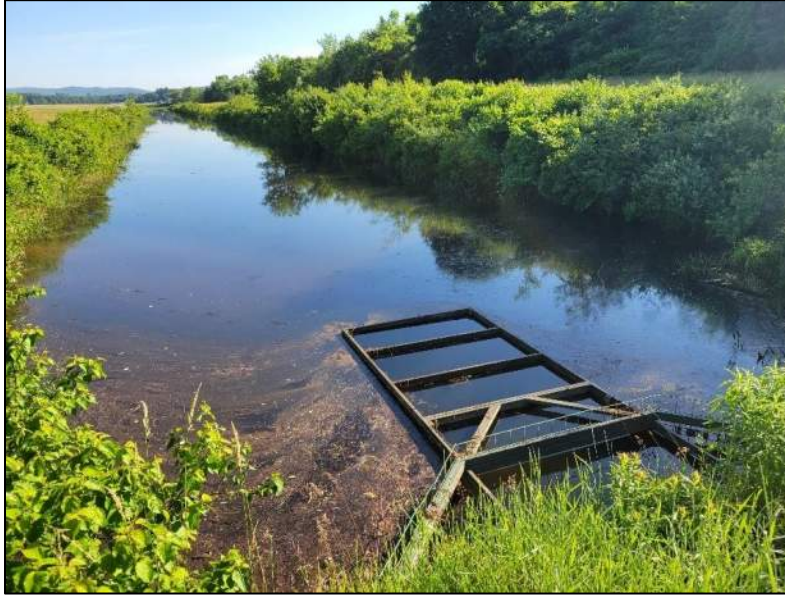
Figure 20. Beaver Deceiver in culvert east of Taxiway Alpha.
