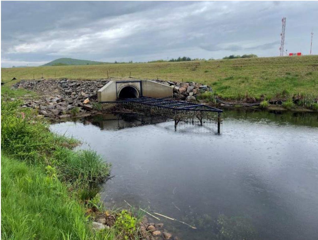
Photo 19: Stream H existing 60-inch RCP inlet on east side of Runway 2
