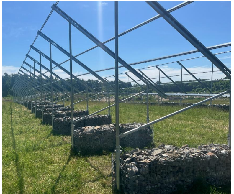
Ballasted array and racking system
