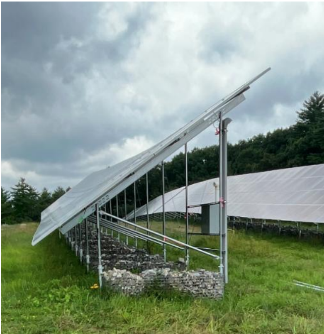
Ballasted array and racking system
