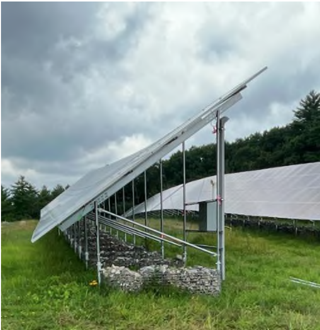
Ballasted array and racking system
