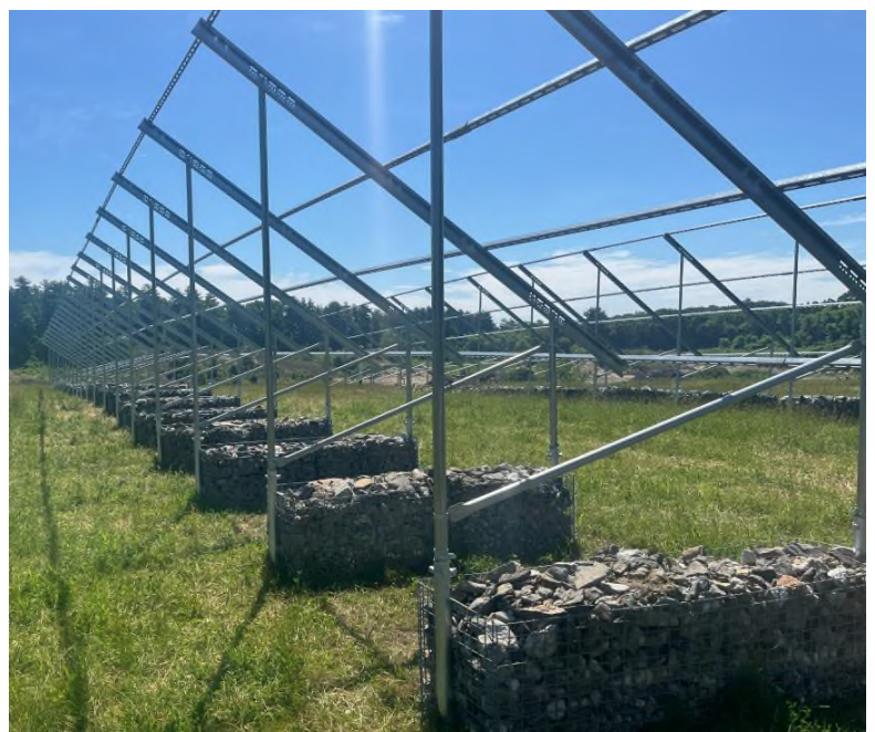
Ballasted array and racking system
