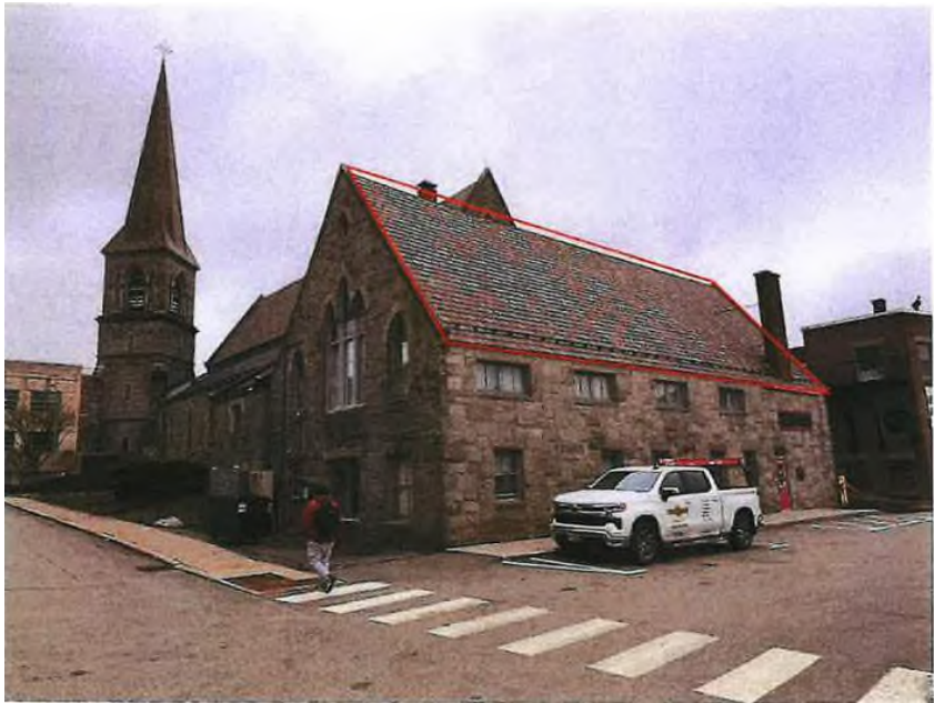
Fig 2: Southern exposure of parish house roof to be replaced for PV system.
