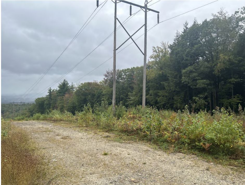
Photo 9 – Proposed Str. 190 work pad, viewing west. (09-24-25)
