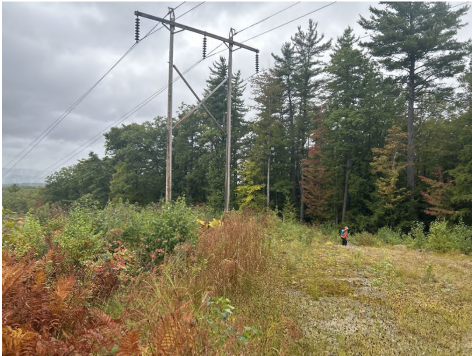
Photo 10 – Proposed Str. 191 work pad, viewing west. (09-24-25)
