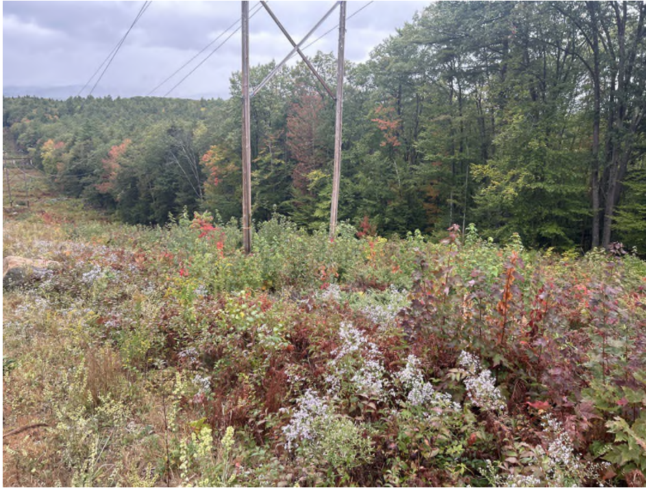
Photo 13 – Proposed Str. 193 work pad, viewing west. (09-24-25)
