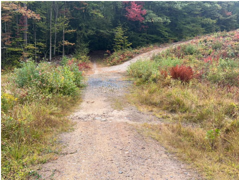
Photo 4 – Proposed wetland crossing of W100 on Old Gilsum Road, viewing north. Existing access road leading to Str. 188 visible on the right side of the photo. (09-24-25)
