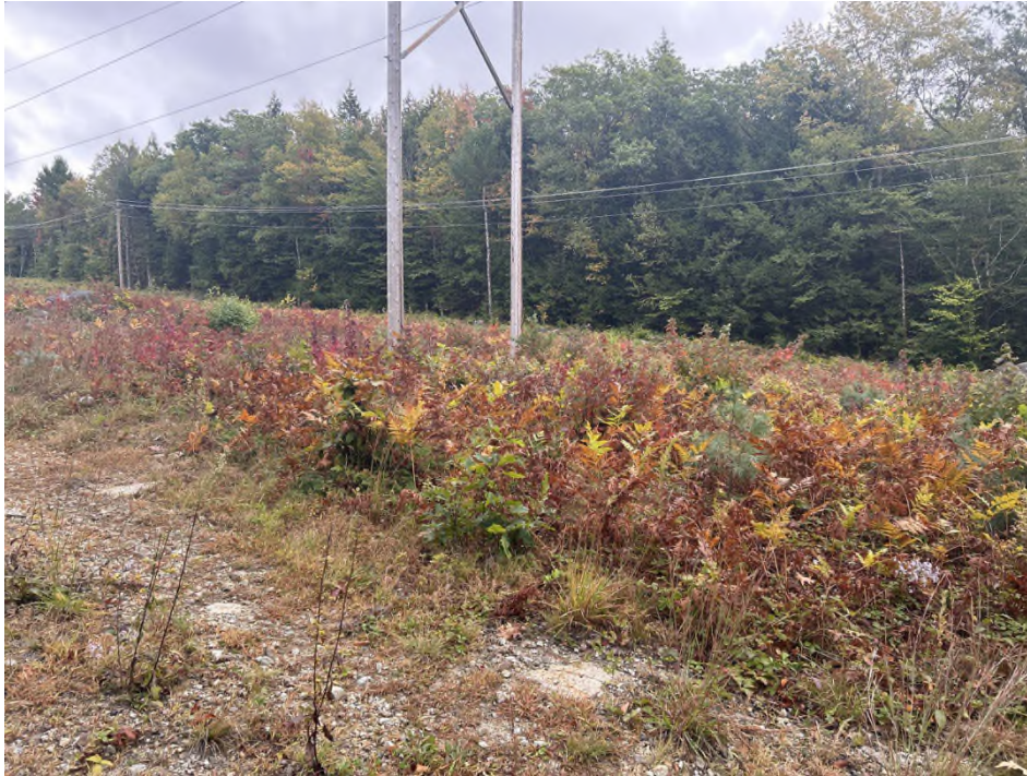
Photo 7 – Proposed Str. 188 work pad, viewing southeast. (09-24-25)
