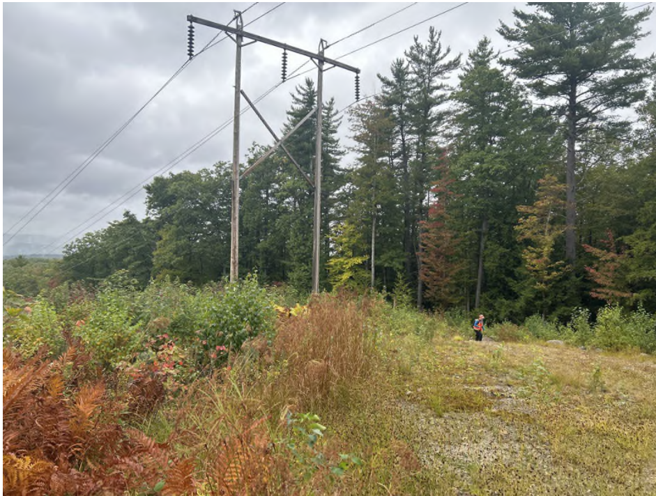
Photo 10 – Proposed Str. 191 work pad, viewing west. (09-24-25)
