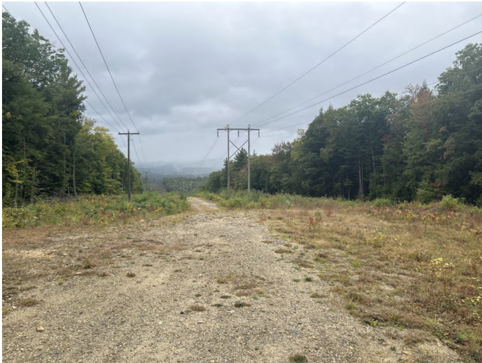
Photo 8 – Overview of the ROW with Str. 190 visible on the right side of the photo, viewing southwest. (09-24-25)
