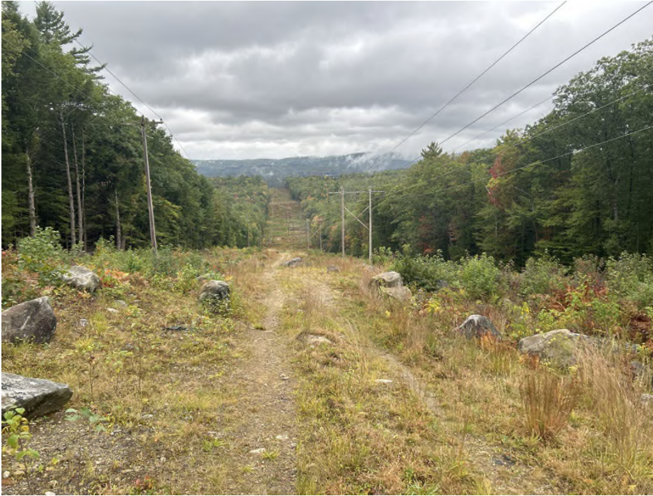
Photo 11 – Overview of the ROW, viewing southwest from between Strs. 191 and 192. (09-24-25)
