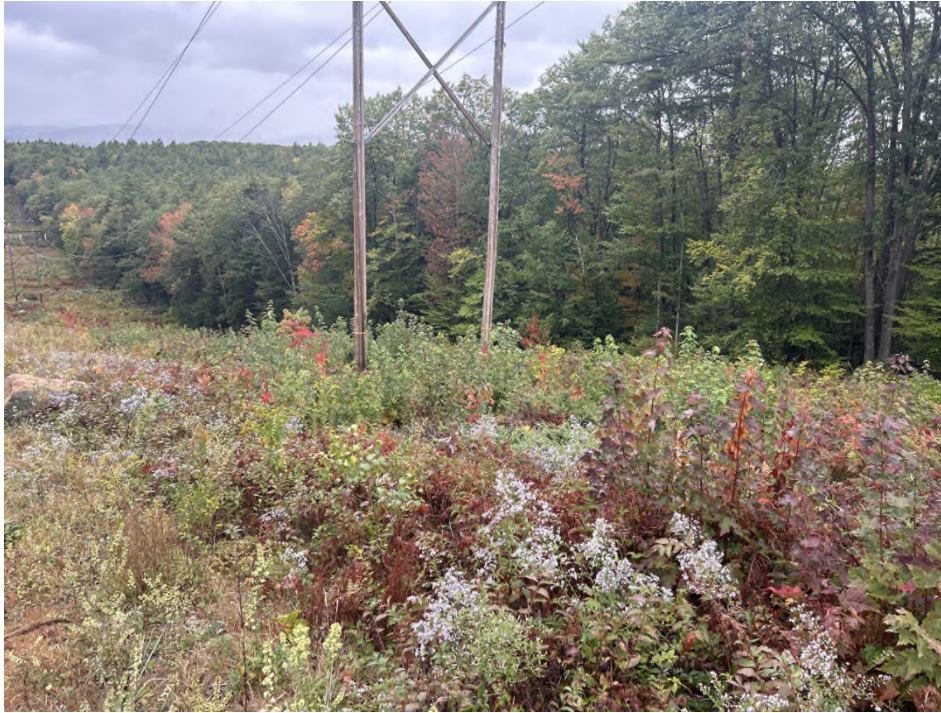
Photo 13 – Proposed Str. 193 work pad, viewing west. (09-24-25)
