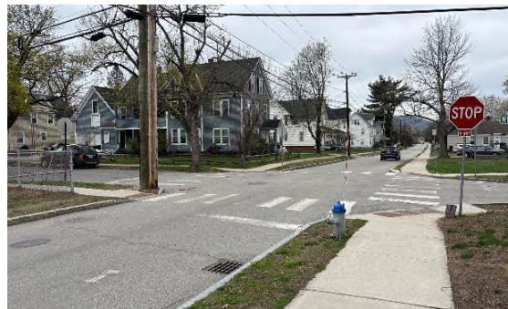
Figure 19. Most downtown area streets (such as the Wilson/Davis intersection above) include sidewalks and crosswalks
