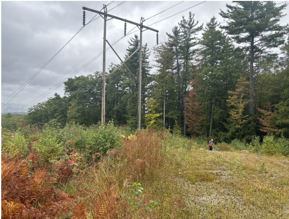
Photo 10 – Proposed Str. 191 work pad, viewing west. (09-24-25)
