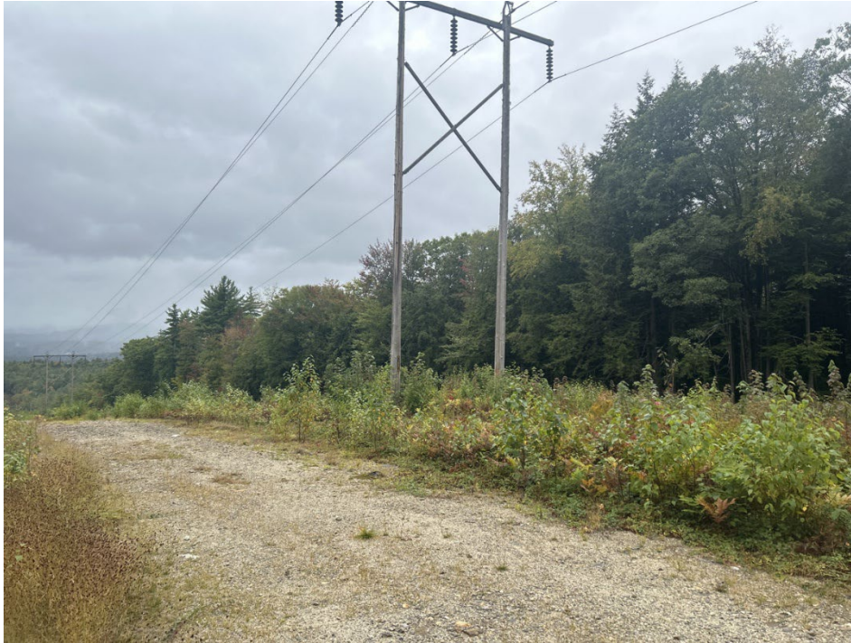
Photo 9 – Proposed Str. 190 work pad, viewing west. (09-24-25)
