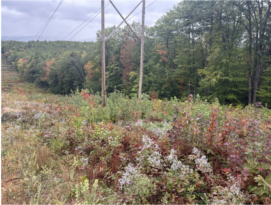
Photo 13 – Proposed Str. 193 work pad, viewing west. (09-24-25)
