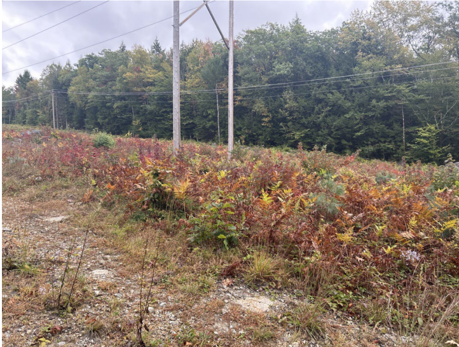
Photo 7 – Proposed Str. 188 work pad, viewing southeast. (09-24-25)
