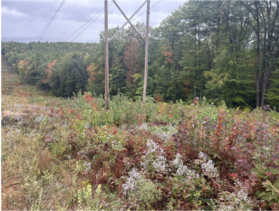
Photo 13 – Proposed Str. 193 work pad, viewing west. (09-24-25)
