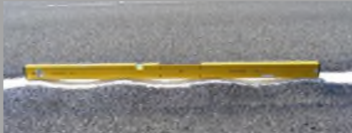
Figure 2. Sinusoidal Rumble Strip - Longitudinal Section
