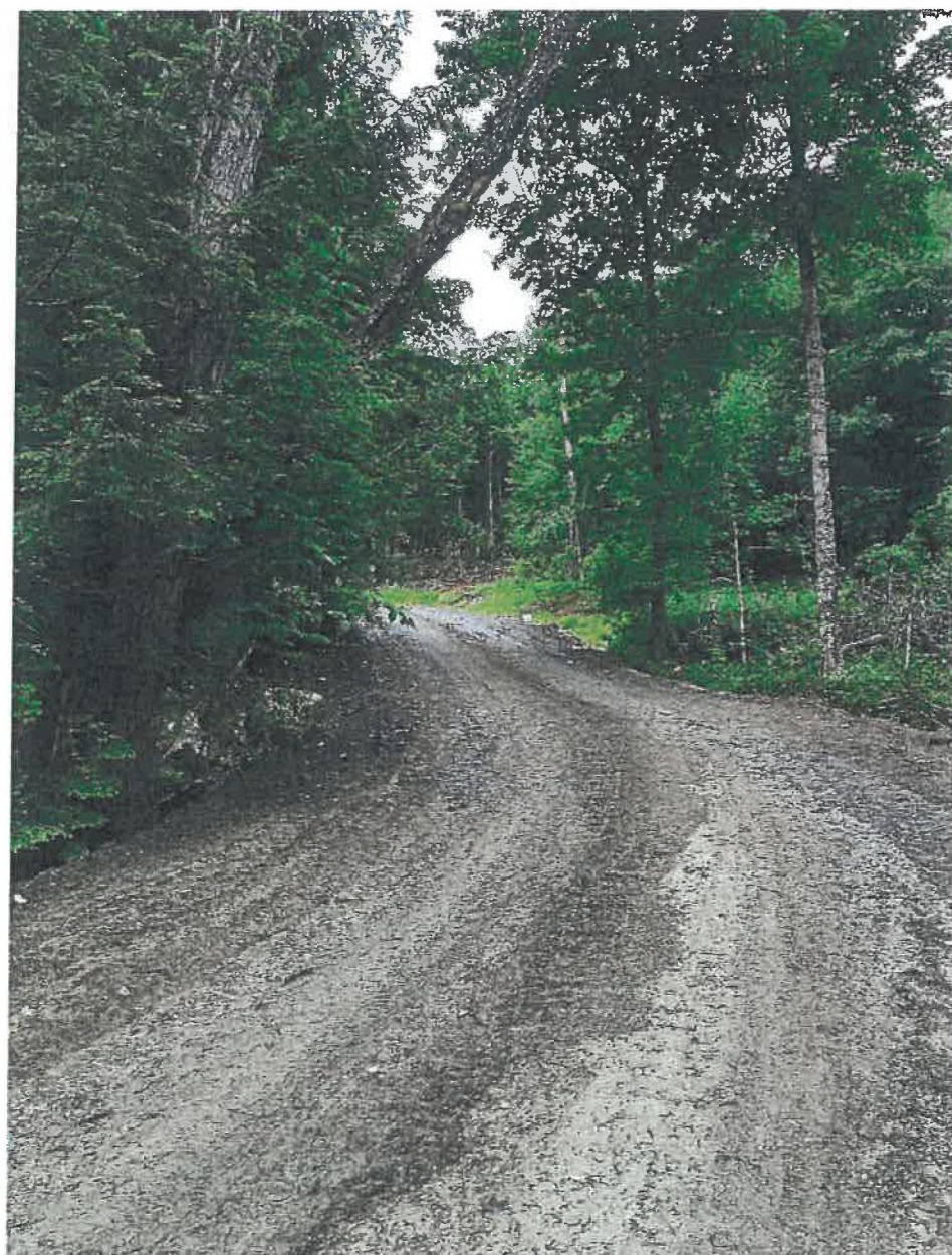
Existing Westerly at Crossing #1 June 11, 2024
