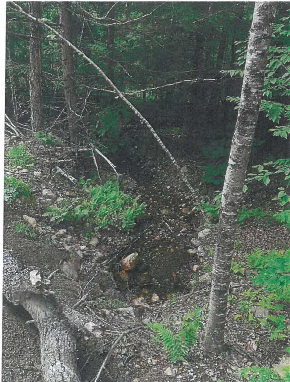
Existing Crossing #1 – Looking Downstream June 11, 2024
