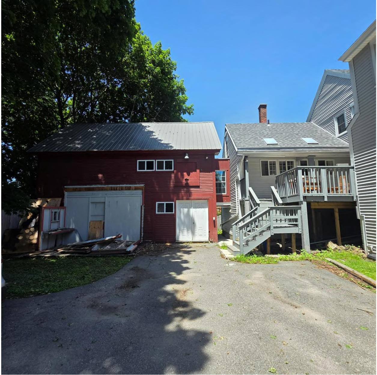
Picture of Barn at the rear of 128-130 School St – South Facade
