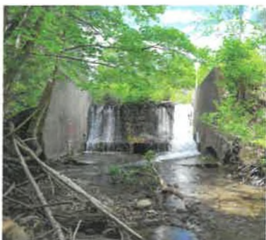
Obsolete dam removal in Springfield, VT.
